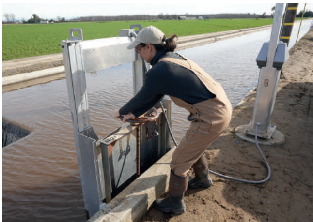
Almond grower Christine Gemperle opens the water supply gate from a canal on her farm to flood dormant almond orchards and perform groundwater recharge using stormwater. Photo courtesy of the Almond Board of California.
