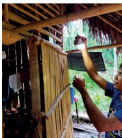
Solar light installation.
